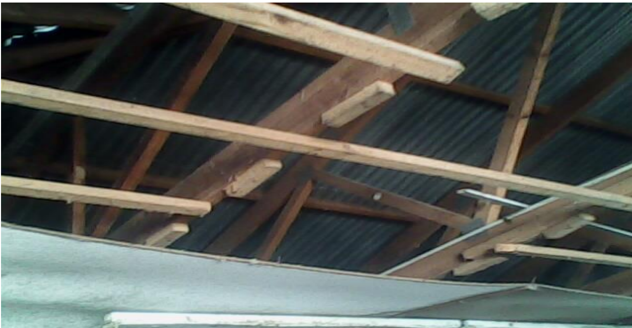
Picture 4: The collapsing roof of the milking parlour at Balu Estate
