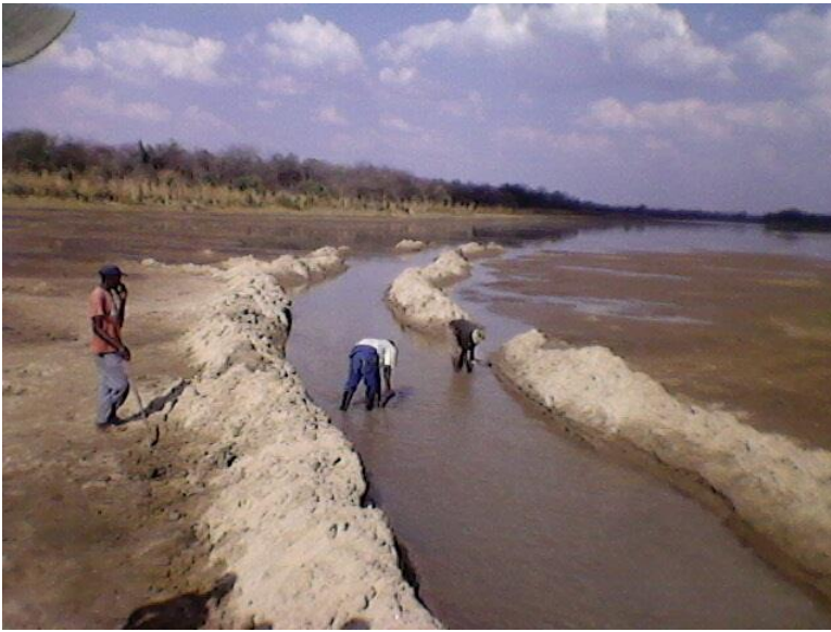
Picture 2: The heavily silted weir at Jotsholo estate
